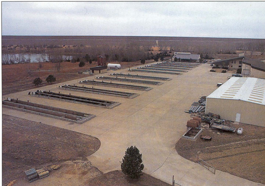
Milford Hatchery, situated below the Milford Reservoir dam, is the state's only intensive hatchery, raising fish in 24 100-foot-long raceways, in addition to six lined ponds.
